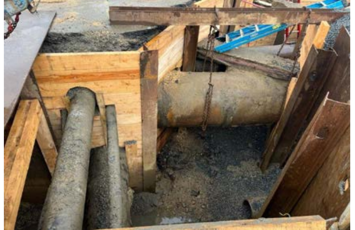
Custom trenching required due to large quantity of utilities in the Lynnway
