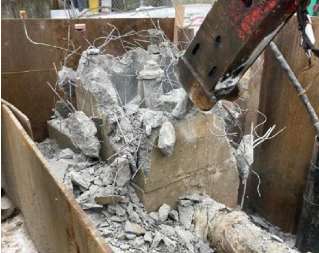
Large concrete thrust blocks discovered in field
